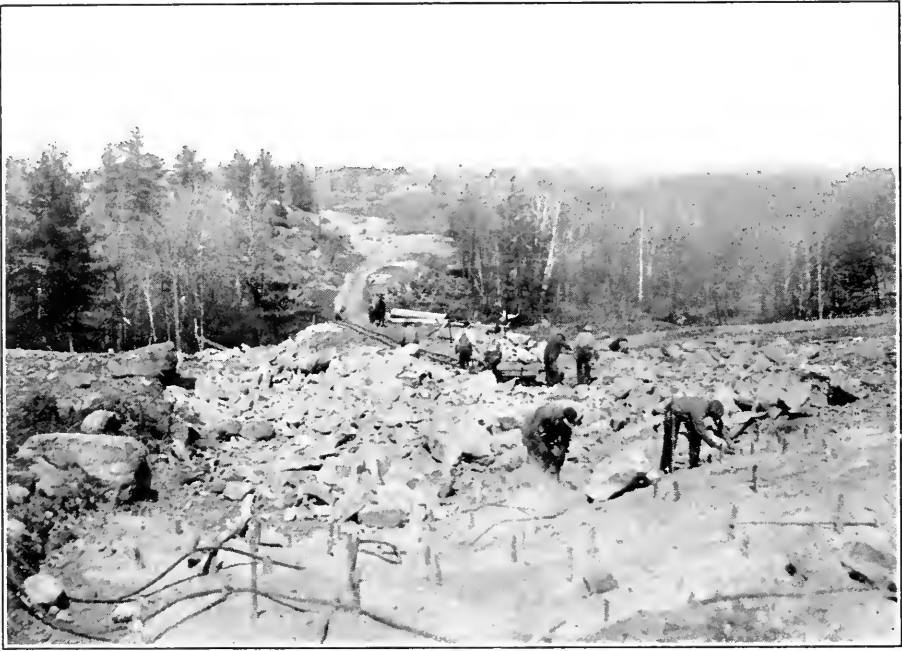
Cut and Fill, Seven Miles South of Kaladar.
